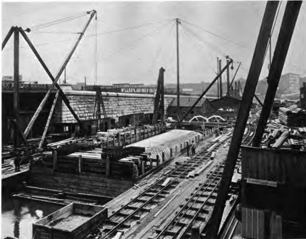
SHOWING CONCRETE OVER IRON WORK — HARLEM RIVER TUNNEL
